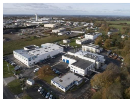
Overview of Sanofi site in Ploërmel
